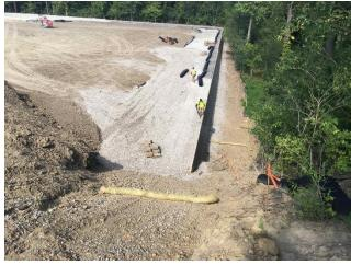
the wall locations, for both top and bottom of wall, to take the setback distance into account, as well as the location of the geopiers. The extent of the geopiers was critical, as there was a limitation on the amount of disturbance that was allowed in regards to the wetlands below the wall near the creek.
