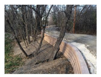
The riverbank provided its own challenges. To prevent excessive environmental damage to the riverbank, all of the construction and access was from the residence side. The use of silt fence during construction, as well as riverbank restoration after construction, had satisfied the environmental damage concerns.
