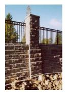
Figure 1: Pillar Block within the Wall Face
