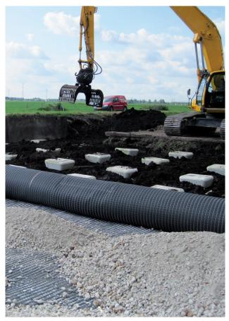
Geotextile reinforcement installed on piles (N 210; Netherlands)
