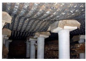
Membrane effect in piled embankment application (Railway Bidor-Rawang, Malaysia)
